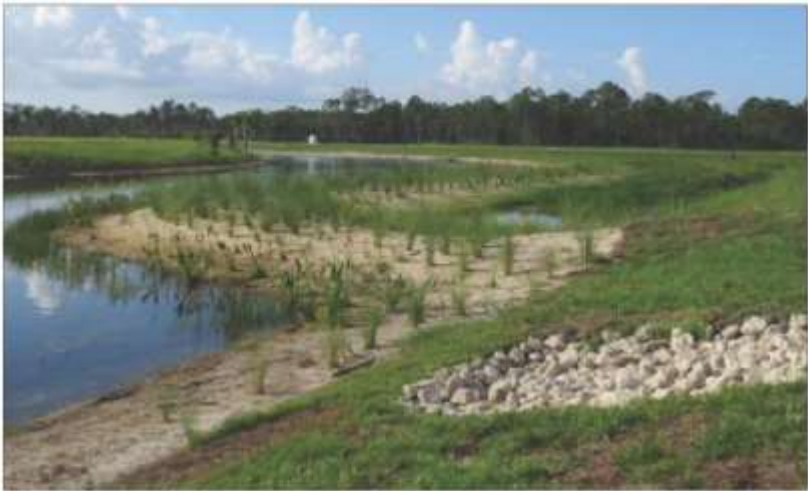
Example of littoral shelves, Diagram of a littoral shelf Image sources Collier County FL.gov
