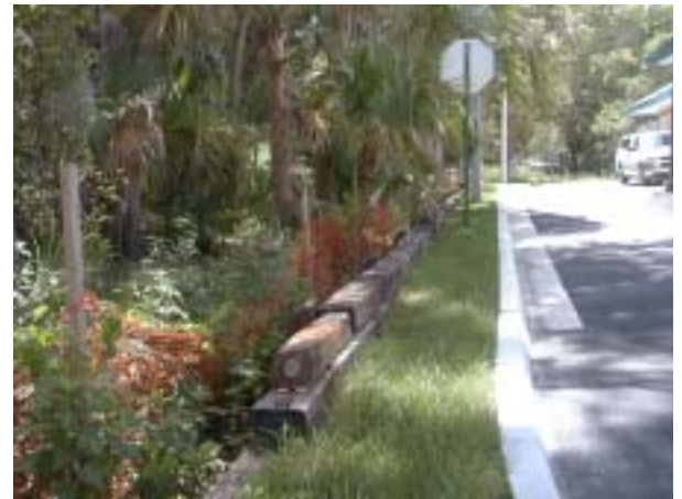
The use of landscape timbers forms a rustic barrier between the paved and native growth areas.
