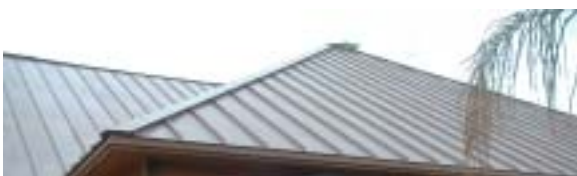
Standing Seam Sheet Metal
