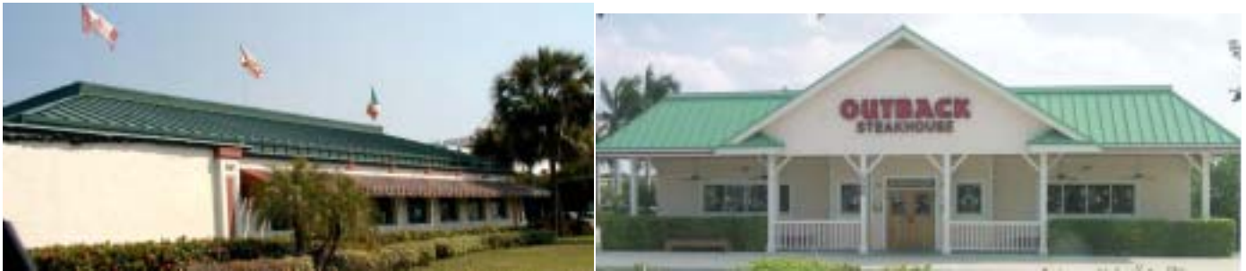
The roofs on these structures are examples of Hip on Deck roof styles.
